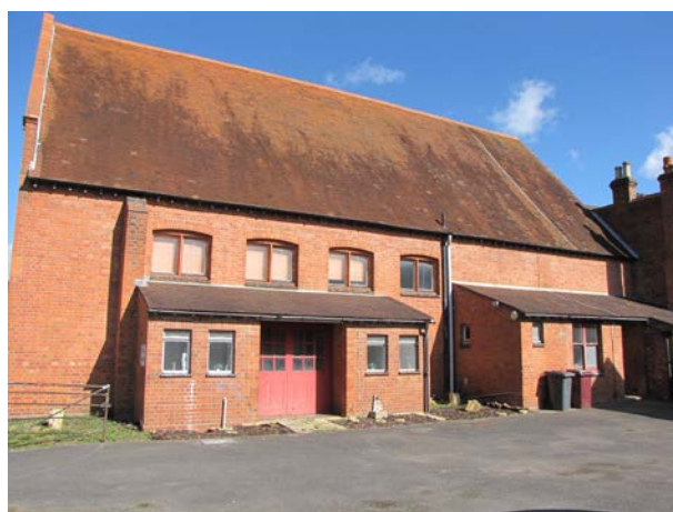
Rear elevation of church
